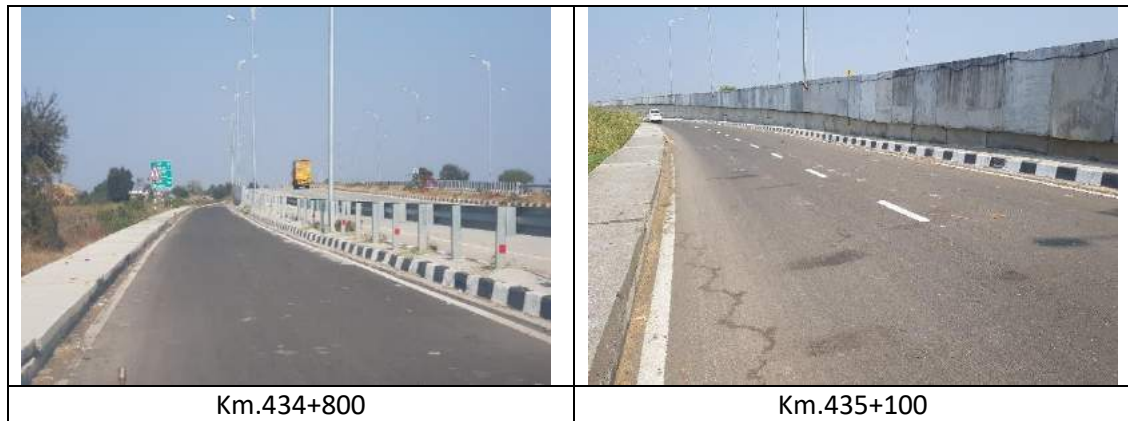
Figure 3-2: Representative Photos of Pavement Condition.
