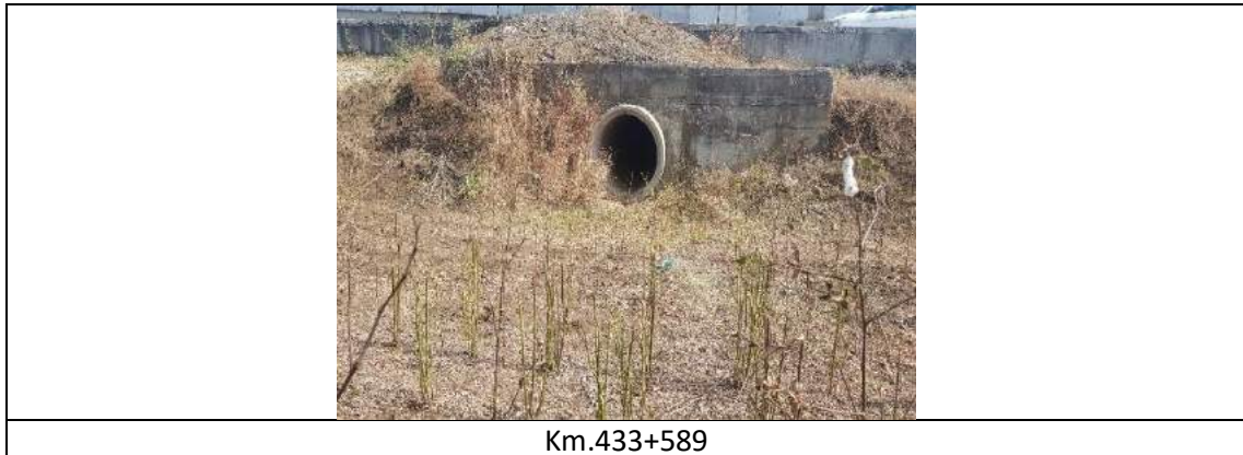
Figure 4-4: Representative photos of Pipe Culverts
