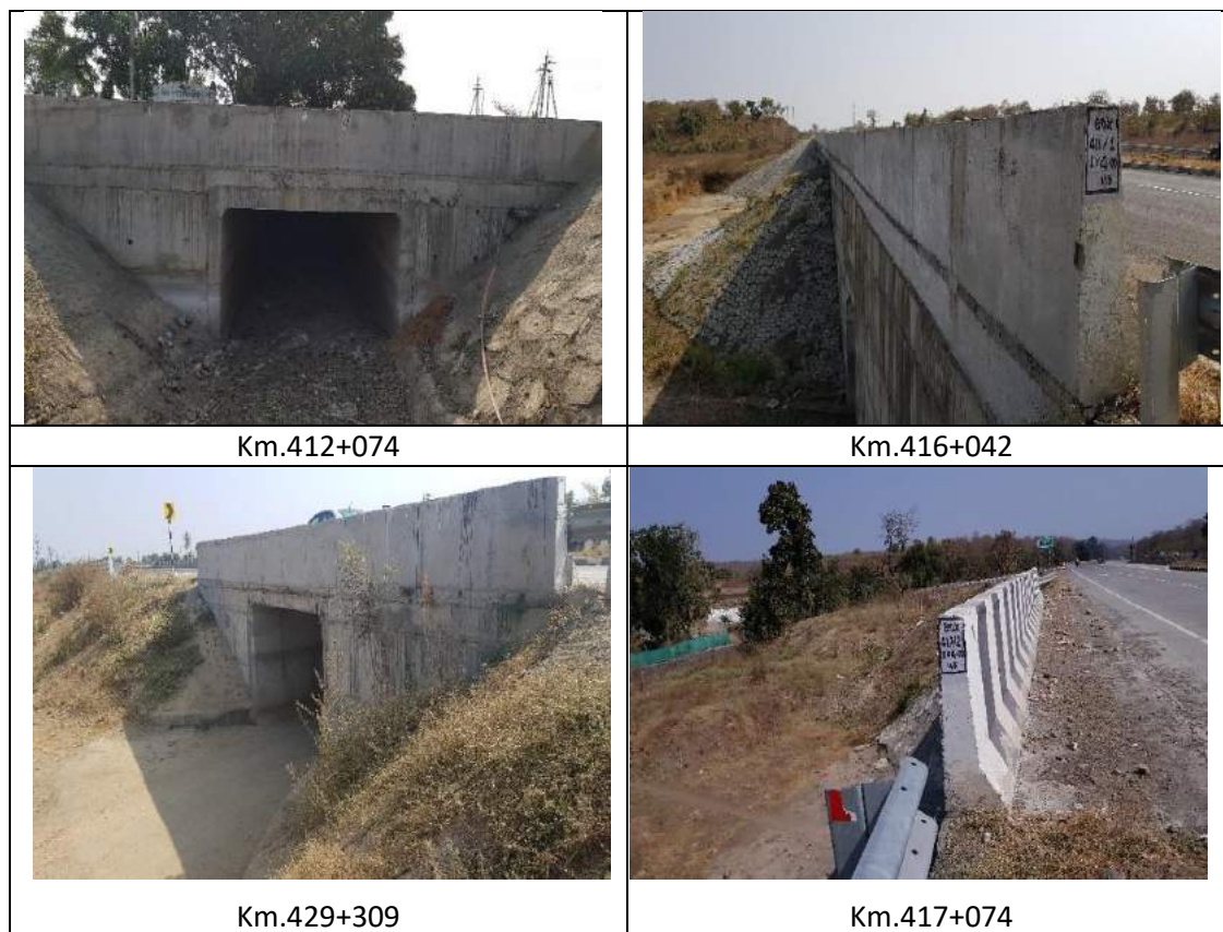
Figure 4-3: Representative photos of Slab Culverts
