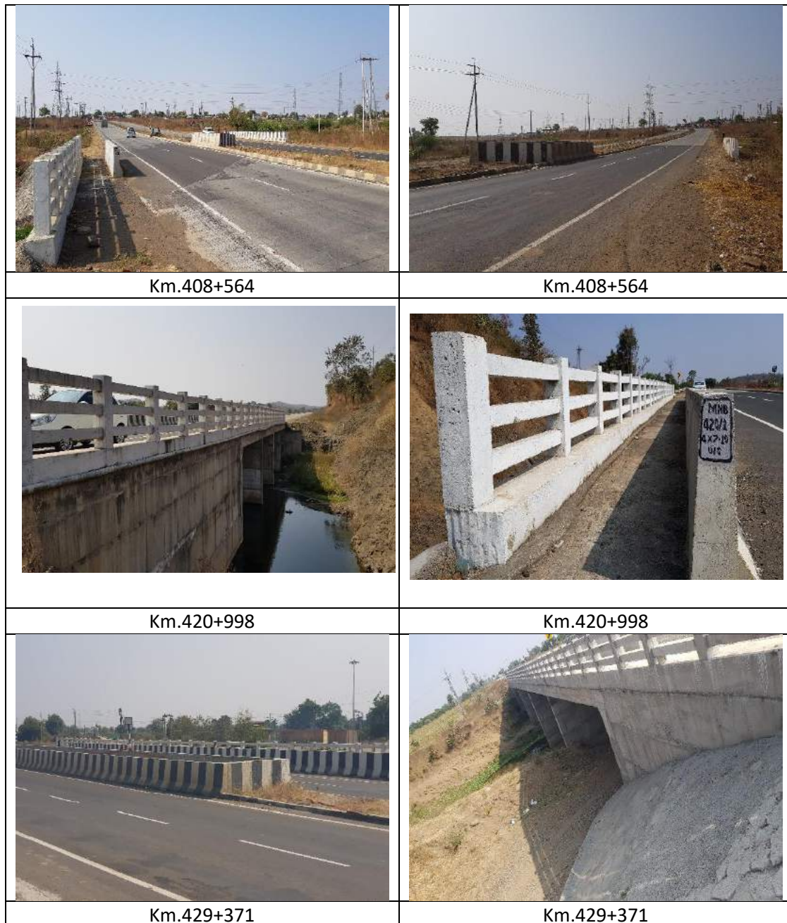
Figure 4-2: Representative photos of Minor Bridges.
