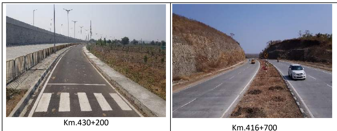
Figure 3-1: Existing Road Features
